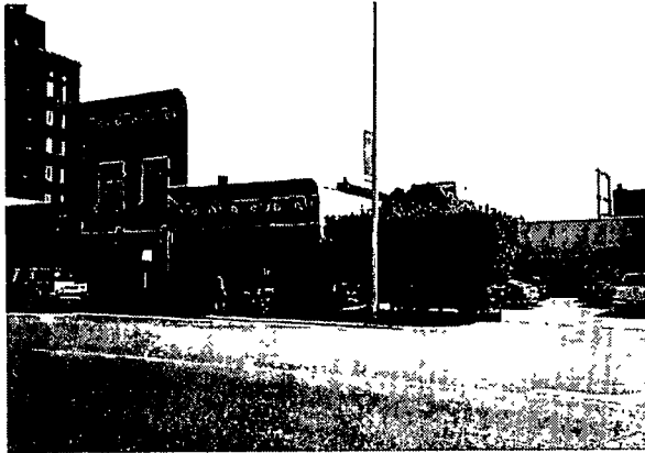
Front Elevation, View Northeast (Photo Taken on September 1, 2015)
