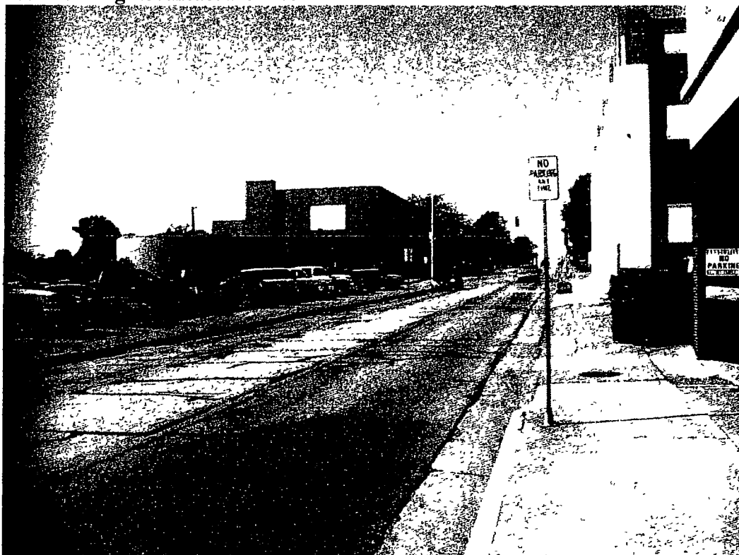
View looking west along north boundary
