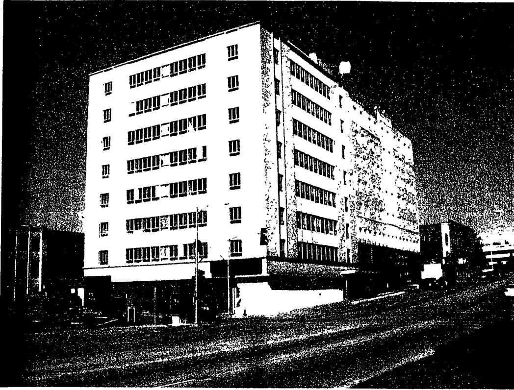
Front view looking N/NW
