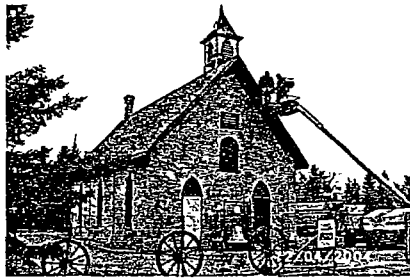
Restoring the roof on Gardiner Presbyterian Church, Battleford, now serving as a community museum
