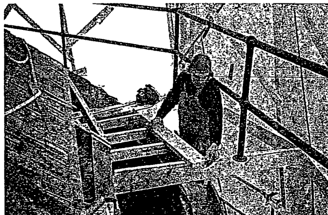
Rebuilding the catwalk on top of the Humboldt Water Tower
