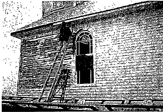
Repainting St. Cunegunda Roman Catholic Church, Horizon
