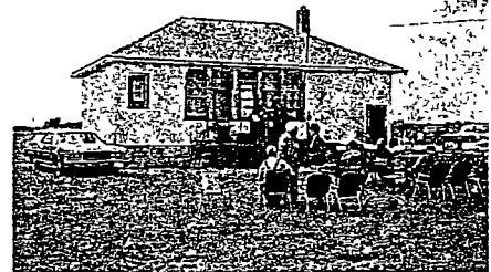
The community gathers to celebrate restoration of the Hayward School roof, near Lipton
